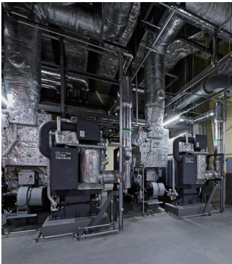
Four of Panasonic’s natural chillers (aka absorption chillers) are responsible for heating and cooling the stadium as a whole.
