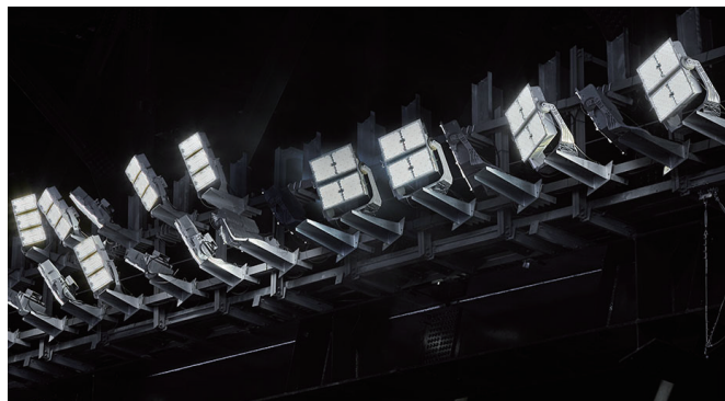
The light direction of each 1 kW/2 kW-equivalent LED floodlight can be adjusted to reduce glare.
